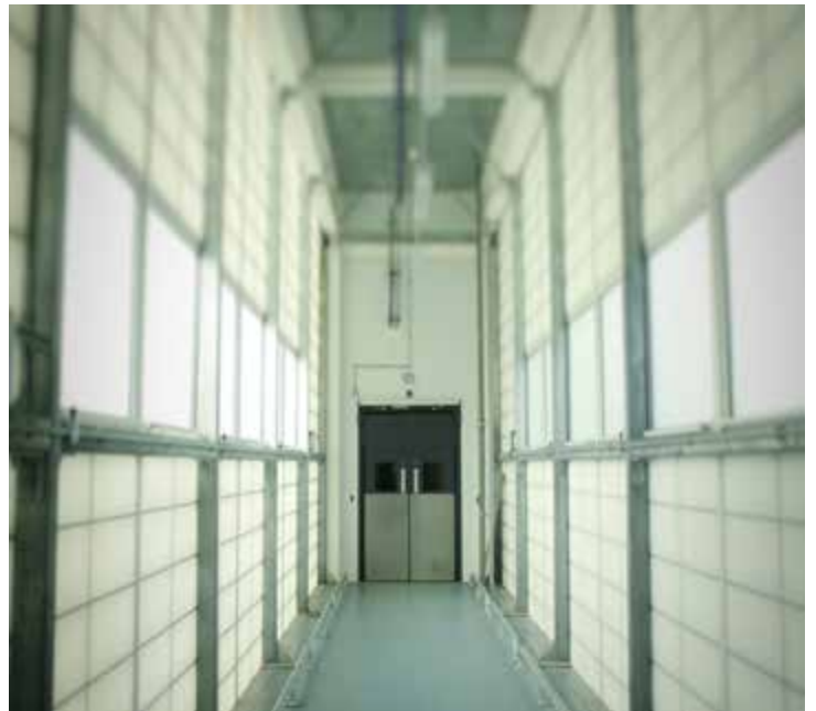
Equinix Data Centre, Slough
